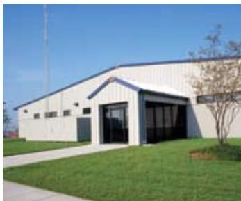
A new shop, service area and hangar in New Iberia are part of a first-class facility in the making.
