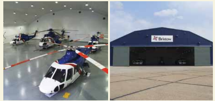
Easily accommodating five S-76s and one AS332L, the new hangar in Norwich, U.K., is enabling better protection for aircraft and reducing congestion in other hangars. An inner skin makes the hangar more functional and durable while allowing for much better insulation.
