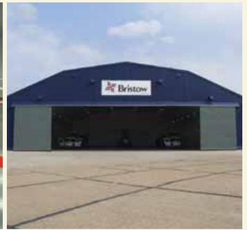
Easily accommodating five S-76s and one AS332L, the new hangar in Norwich, U.K., is enabling better protection for aircraft and reducing congestion in other hangars. An inner skin makes the hangar more functional and durable while allowing for much better insulation.
